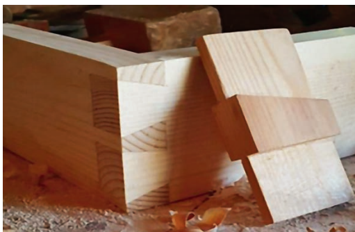
Figure 13 Through dovetail, 1:5 ( https://tinyurl.com/261yt3am )
