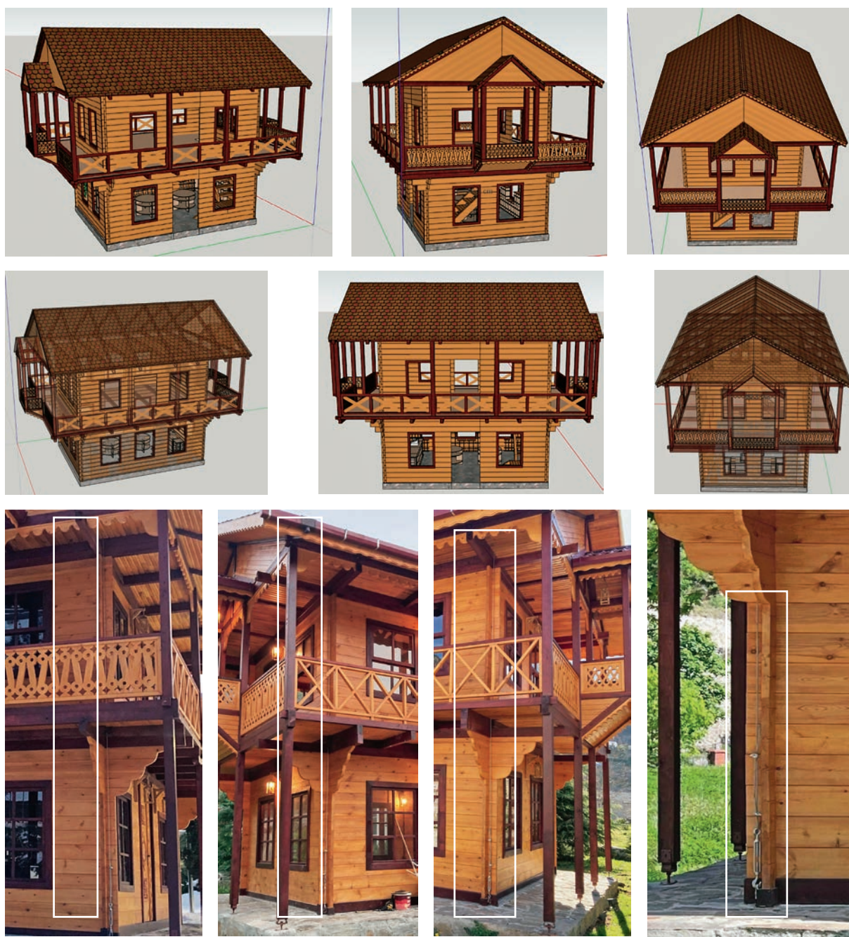
Figure 2 Some images of 3D views and grooved joints (white rectangular)
