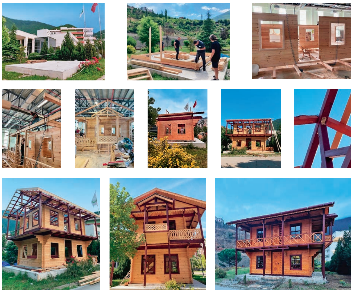
Figure 1 Some images of construction stages
